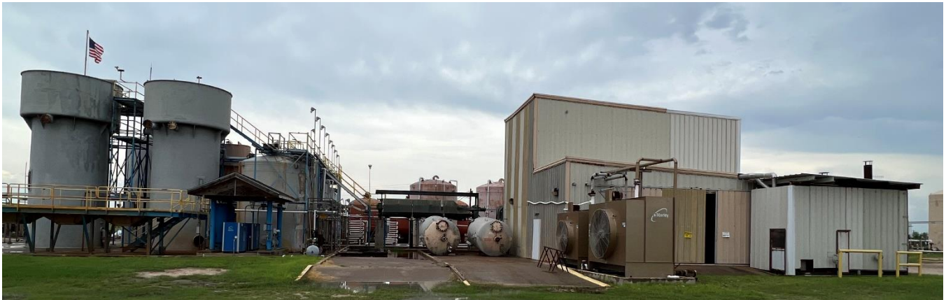
Figure 14: Kingsville Dome Processing Plant
