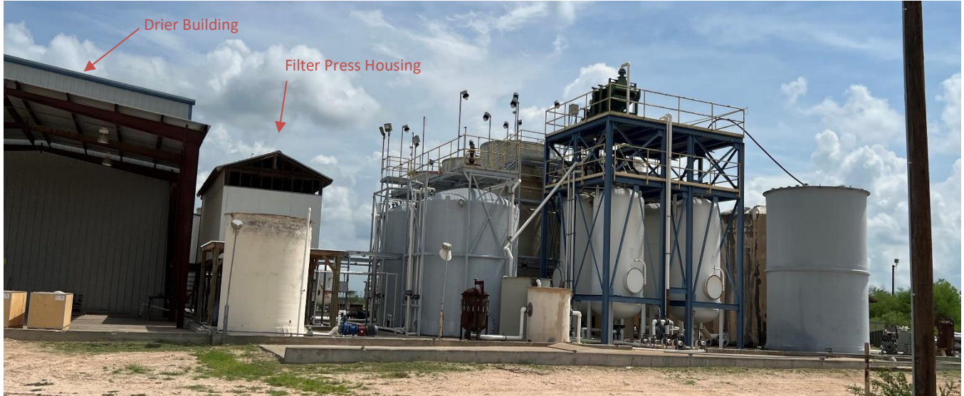
Figure 2: Rosita Plant at Ground Level (Aug. 30 th , 2022)
