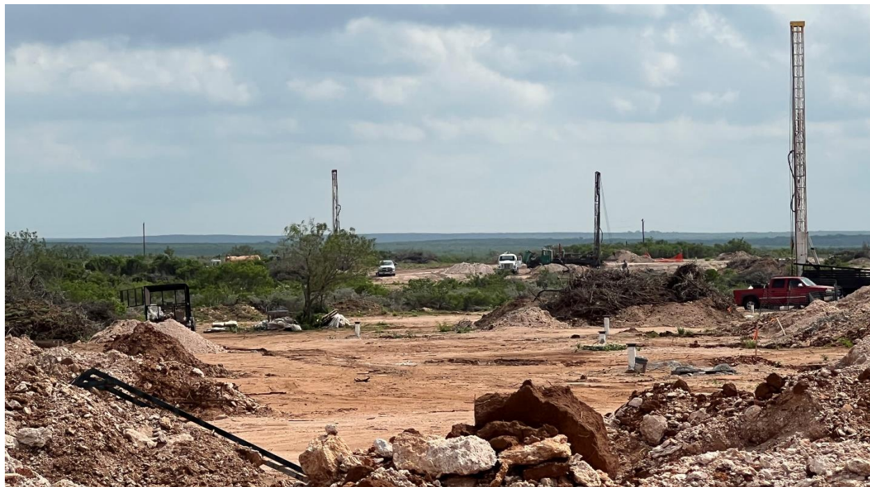
Figure 10: Highlighting a very active Rosita Extension PAA site with multiple drill rigs at work
