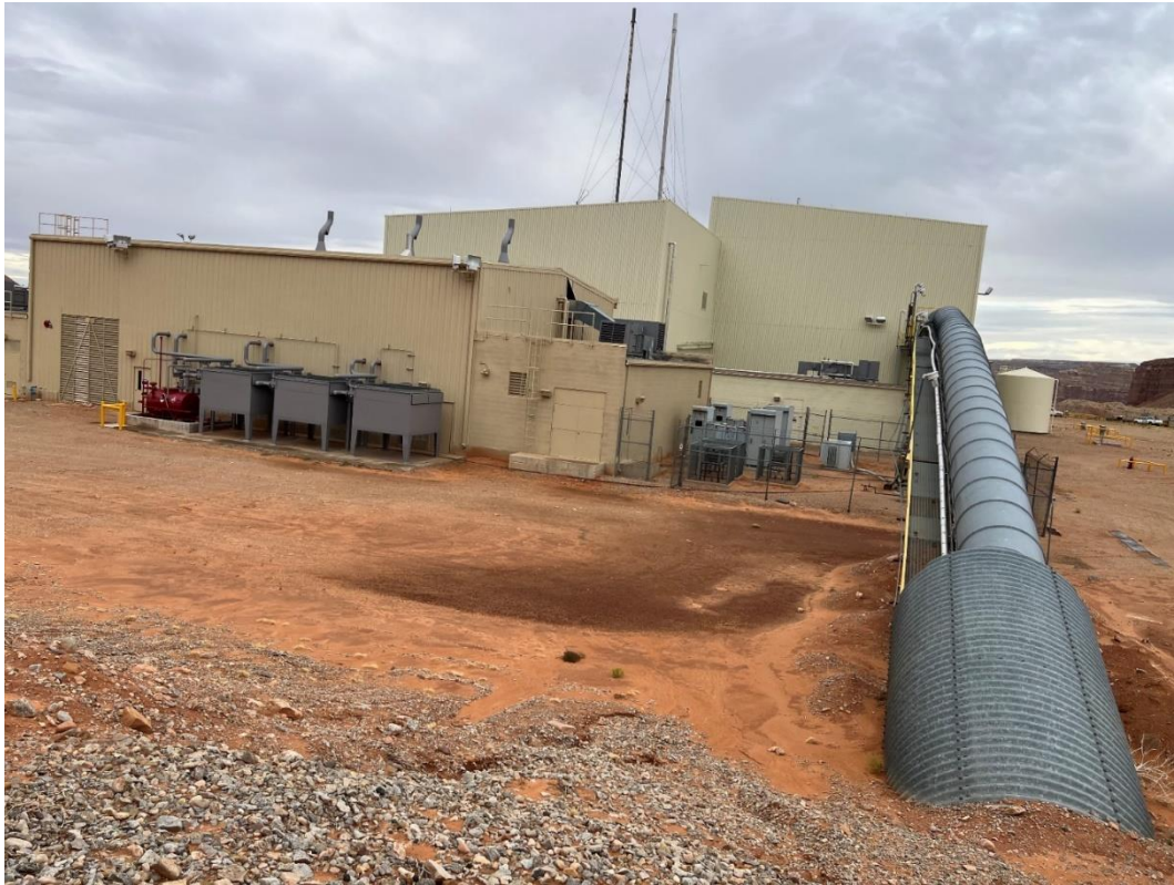
Figure 4: Upper/Lower: RoM conveyor covered housing to mill – Conveyor is in very good state of repair and should be turn-key
