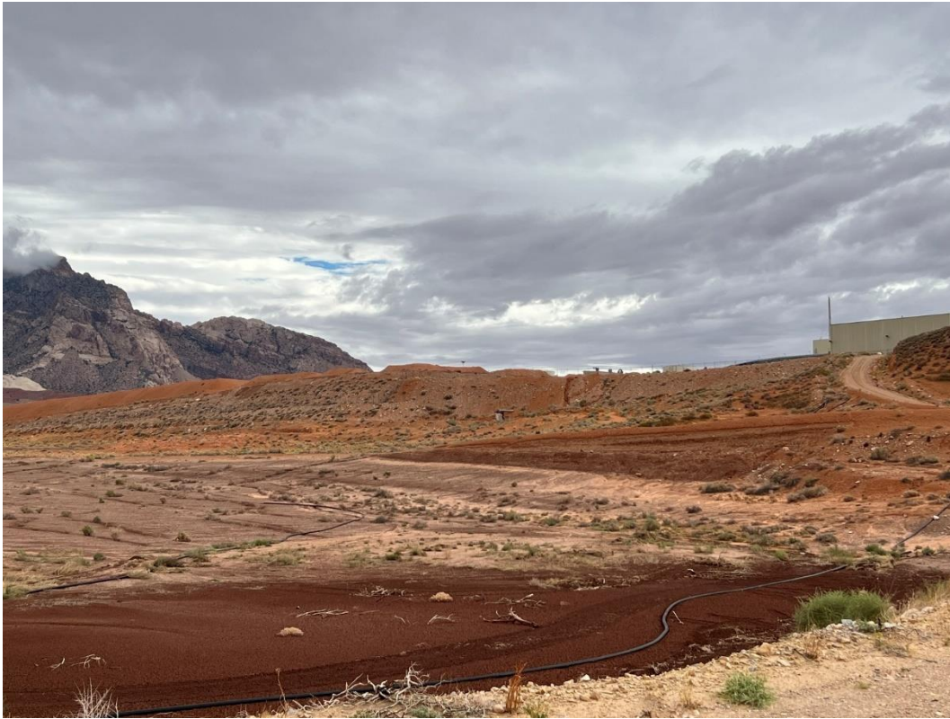
Figure 10: Upper/Lower – standing on 80-acre tailings area (mill visible in upper picture at right). Refurbishment of the tailings area will involve modern spec linings being installed. Capacity is ample and expected support decades of processing.
