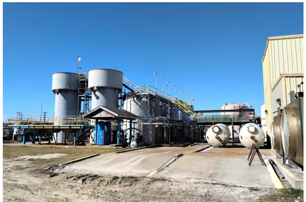
Photo 1: Kingsville Dome ISR plant site showing various ion exchange, elution, precipitation and reagent storage tanks, filter press (covered in green wrap) and adjacent dryer building.
