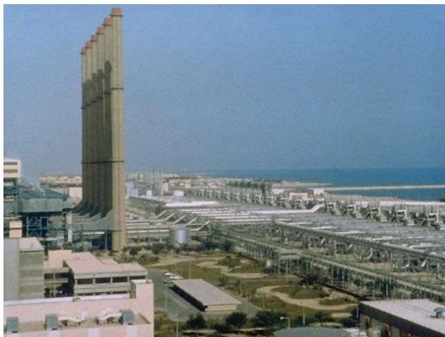
Saudi Arabia's Jubail desalination plant is the largest in the world, daily converting 800 million gallons of seawater into much-needed fresh water.
