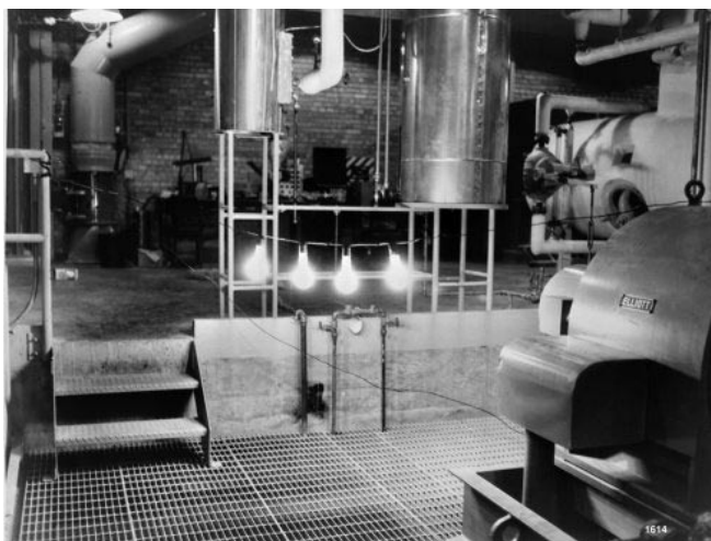
Four light bulbs were lit with America's first civilian nuclear reactor in 1951, capable of producing electricity. Courtesy: Idaho National Laboratory
