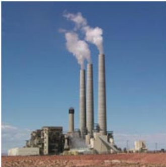
The Navajo power plant: a coal-fired, electric-power-generation plant near Page, Arizona (USGS)
