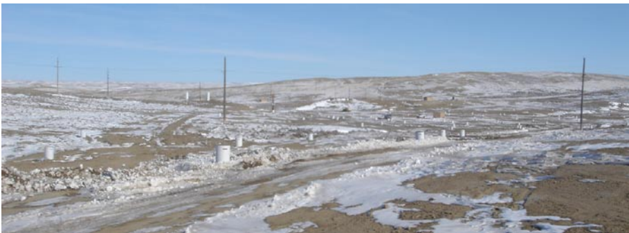
Cameco Corporation's Smith Ranch In Situ Recovery well field (production and injection wells) in Wyoming (February 2006)
