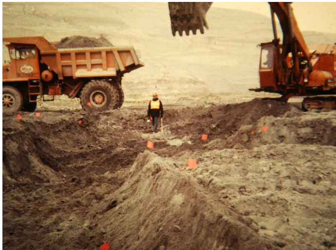
A scraper digging a trench for an open pit uranium mine in Wyoming in the 1950s
